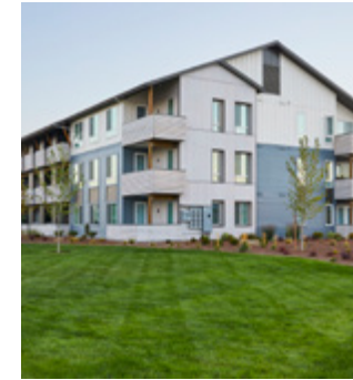
207 East - Edgewood, WA - Drywall & Paint Supplementation, Punch, ADA Compliance Items
